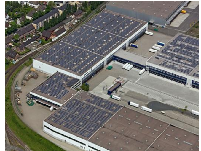
Kühne + Nagel Duisburg, Germania 996,36 kWp (2010)
